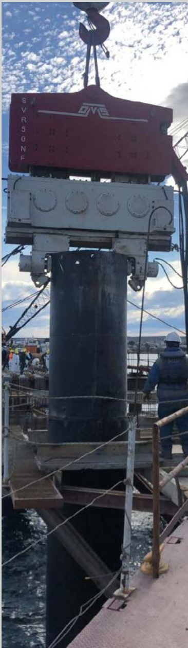
Crane Suspended Pile Drivers
